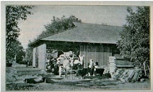
Fig. 2.—Sidwell drying house, outer walls made of slats to give good ventilation.
