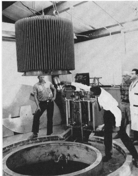
A seven-ton lead "pig" containing the Cobalt-60 is being lowered through the roof into the pool. Exposure readings are taken by the Radiation Safety Officer.
