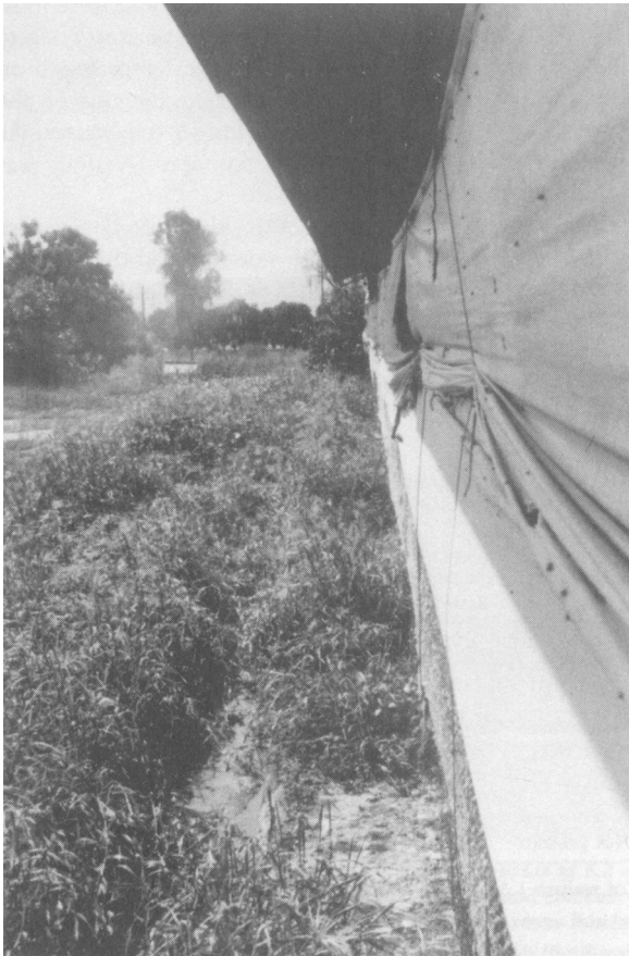
Fig. 9. K2 egg ranch south wall in August 1983. Note water accumulation at drip line and weed growth.
