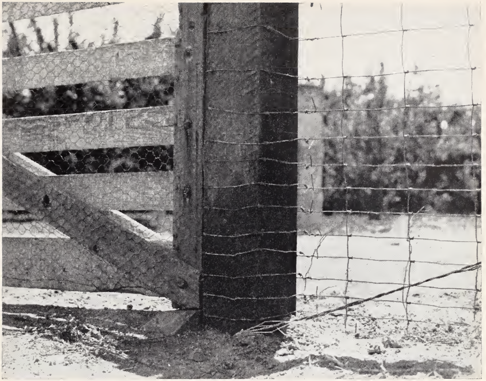
Fig. 25. Rabbitproof fence and gate. Bottom of fence wire is buried 6 inches or more and lower meshes should not be more than 1\frac{1}{2} inches apart. Gate is covered with 1-inch poultry netting and bottom of gate must be within 1\frac{1}{2} to 2 inches of the ground.
