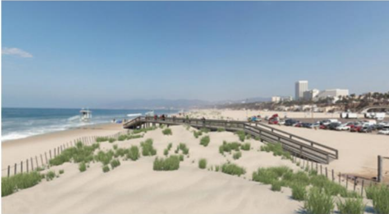
Sand dunes as an adaptation measure to respond to wave run-up due to SLR
