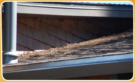
Accumulated pine needles on this complex roof could allow embers to to ignite roofing materials.
