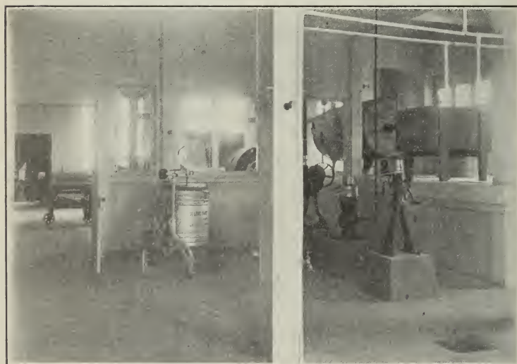
Creamery—Separator and Churning Rooms.
