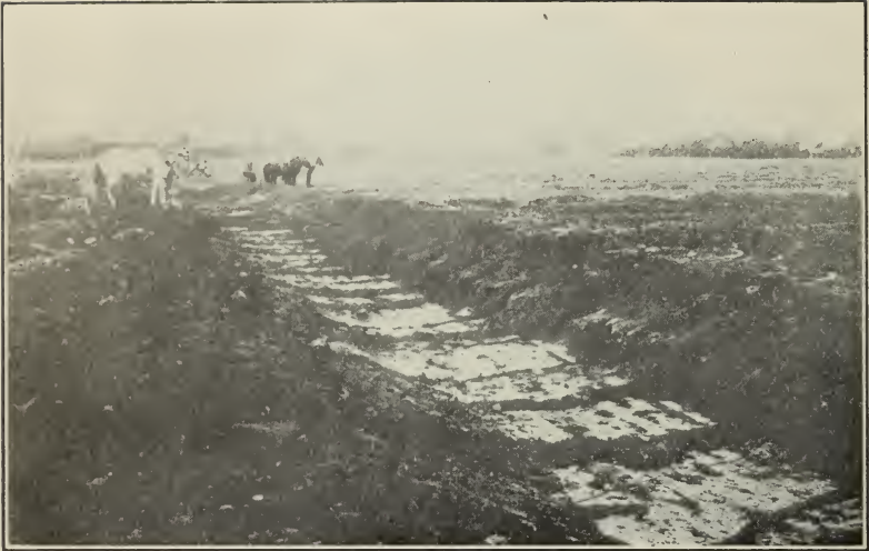
Constructing an irrigating ditch.
