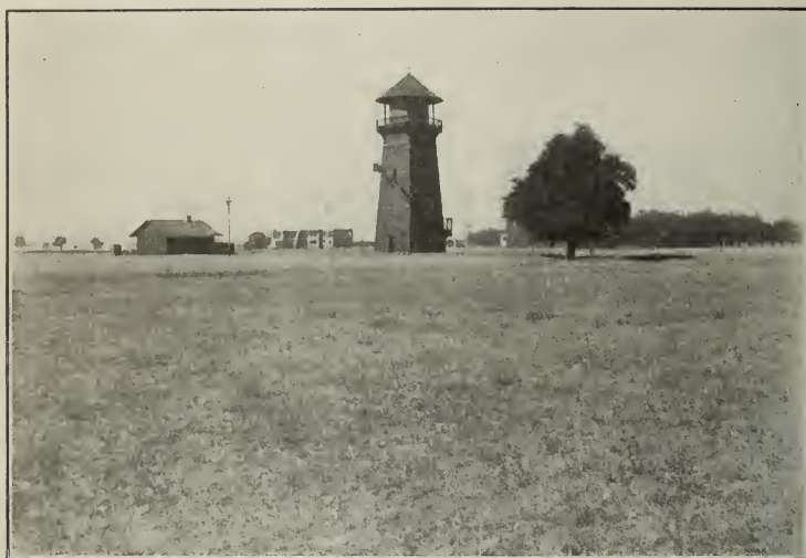
Cottage No. 2 and water tower. Dormitory under construction in background.
