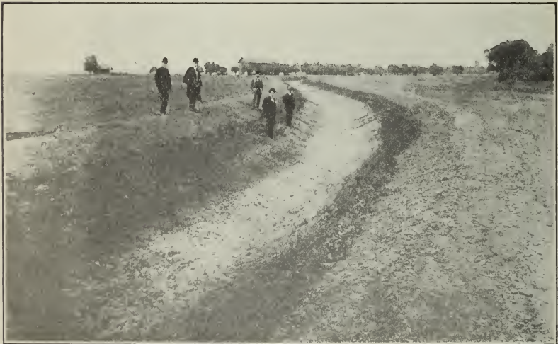
The completed irrigation ditch.
