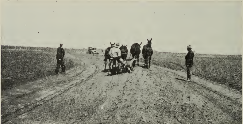
Fig. 28.—Putting the finishing touches on a broad-base terrace. Such a terrace is very little obstruction to cultivation.
