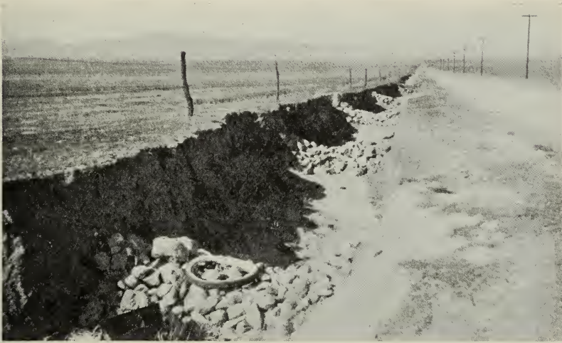
Fig. 32.—Cobble check dams in a roadside ditch which threatened to become a serious menace. This is a more permanent check than the one shown in the preceding picture.
