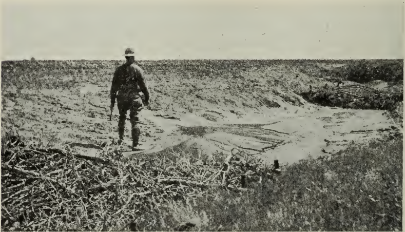
Fig. 31.—Brush soil-saving dams are used not only to prevent gullies from becoming larger but also to collect and retain the soil so that they are gradually eliminated. After the brush becomes firmly imbedded in silt, the accumulation behind the dam becomes very rapid.
