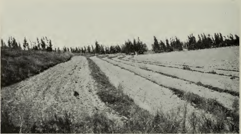
Fig. 26.—Bench terraces near Greenfield. No erosion has occurred on this rather steep slope since the construction of these terraces. Note that the native grasses are allowed to grow undisturbed on the risers.
