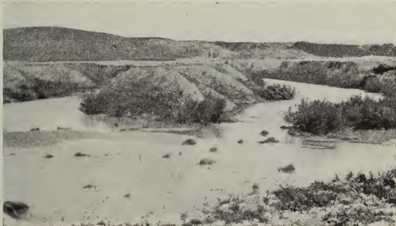
Fig. 37.—An earth dam, a portion of which shows in the lower right-hand corner of the photograph, was constructed across this deep forked gully. The gully is now being gradually silted up and may sometime be tillable land. How much easier it would have been to have taken similar precautions when the gully was only a foot or two deep!
