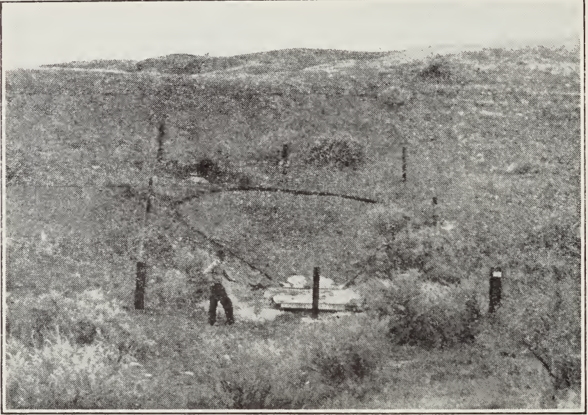
Fig. 21.—General appearance of the watering device of figure 20 as installed. The 3-strand barbed wire fence excludes domestic livestock. (Kettleman Hills, Fresno County.)
