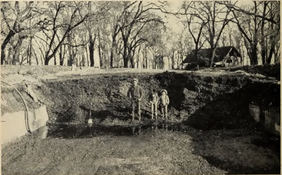
A trench silo partially filled with almond hull silage. This trench is 30' x 175' x 11' and is located on the Roney Brothers Ranch, in Butte County, California.
