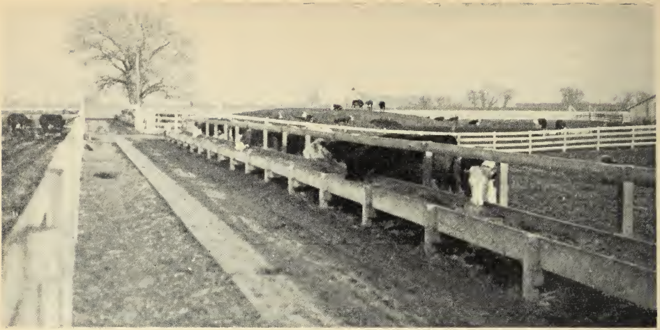
Fig. 34 (V). An economical type of feed-bunk construction for convenient feeding of silage, cut mixtures, wet beet pulp, or wet brewers' grains. In the right background is a mound built to reduce muddy feed-lot conditions.
