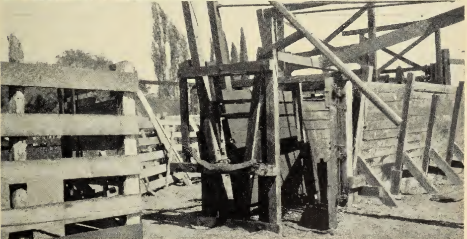
Fig. 31 (IV). This cattle chute and squeeze is adapted from what is known as the Nevada low-cost dehorning chute. The body squeeze and neck squeeze operate as in other types of chutes. The distinguishing feature is the absence of a front exit; the animals leave the chute through one side which is hinged and operated as a side gate.
