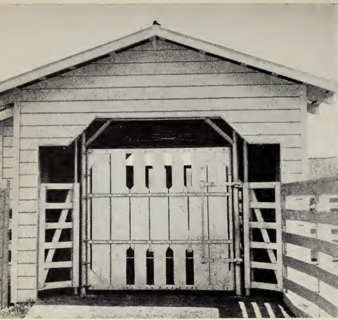
This scale house was built over the scale and rack. One disadvantage of such a house is that the scale rack cannot be removed for weighing trucks or other large equipment.
