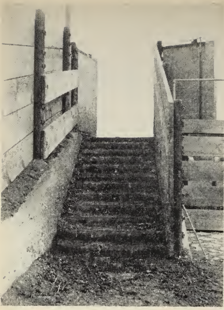
Stepped-ramp loading chute. Steps should be at least 18 inches wide, not over 4 inches high.
