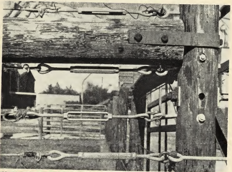
Cable tighteners. To keep cattle from loosening cables, a nut should be placed at end of screw eye. On 5' posts, cables are 9" apart with lowest 12" off ground.
