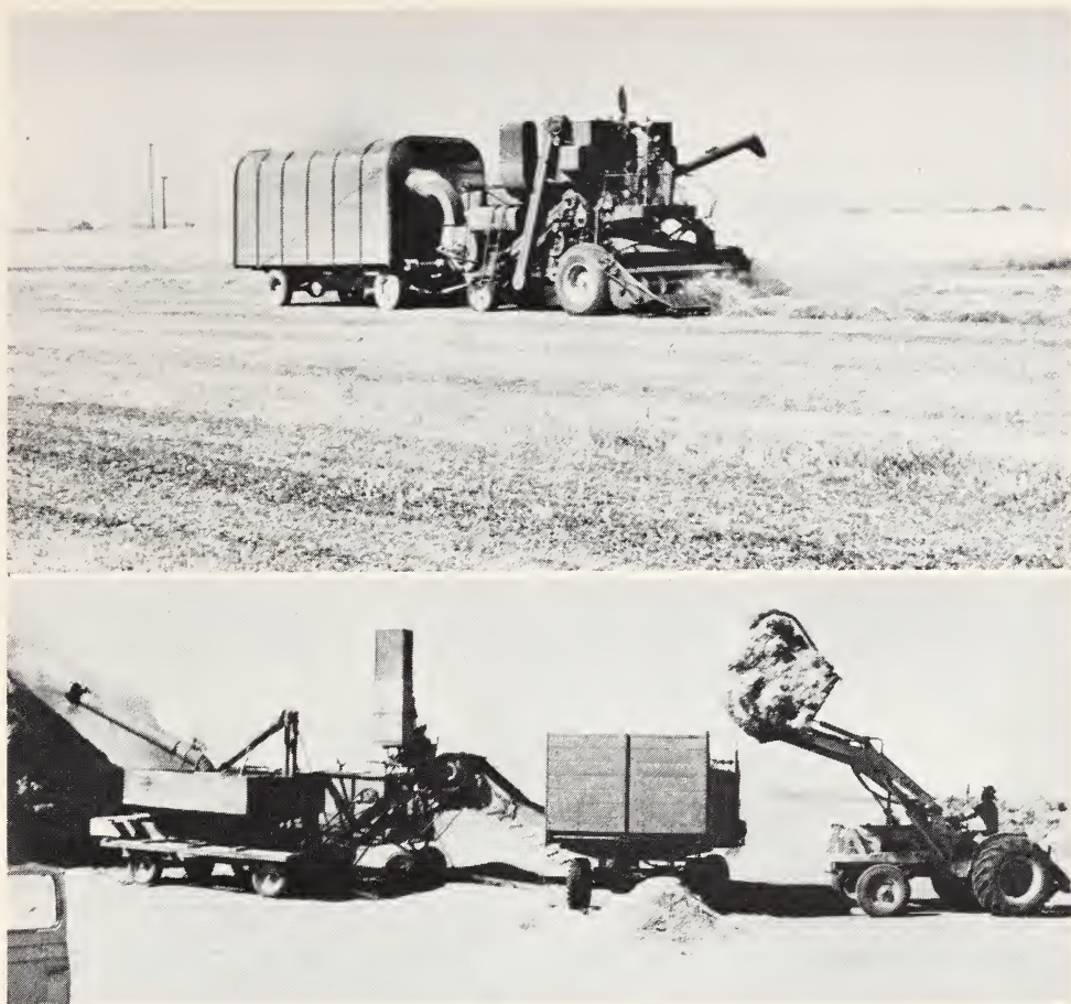
Fig. 34. Combining from windrows with a self-propelled harvester (top), and collecting straw and chaff for rethreshing (bottom) with a stationary thresher.
