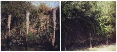
Hog-wire and chain-link fences at the base of cut banks reduce stream velocity and collect floating debris, further absorbing erosional energy. Seedlings become established at the base and lower slopes of cut banks behind the fences.
