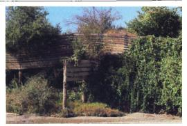
Wooden fences built along lower Dry Creek in earlier years effectively protected cut banks. They were often 3 to 6 meters tall, over 50 meters long, and constructed with largedimension lumber.
