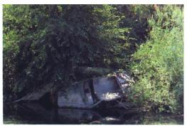
Car bodies, often in four or five tiers, are laced together by cables in stacks as long as 100 meters against cut banks. Sediment collects inside, providing a substrate for tree growth. In older stacks, only 20 percent of the car body surface is now exposed.
