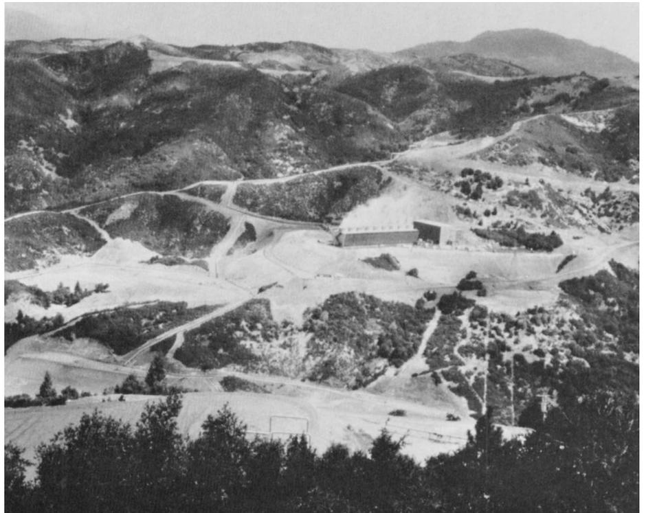
Geothermal power plants (above and opposite) with the associated site disturbances by drill-pads, steam transmission lines, roads, and electric power at The Geysers, northern California. (Photos by Craig Martz.)
