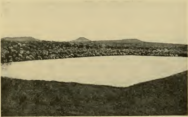
FIG. 113.—AN EARTH RESERVOIR IN NORTHERN ARIZONA BUILT TO COLLECT AND CONSERVE FLOOD WATER FOR WATERING SHEEP.
