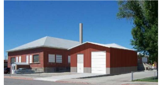
Boiler house and School, Ely NV
