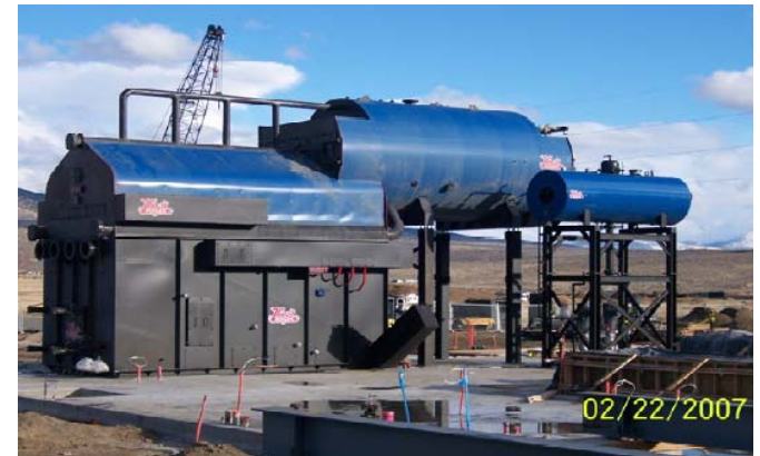
Boiler Installation, Correctional Facility, Carson City, NV
