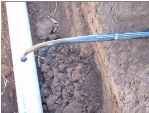
Figure 6: Drip tape laterals were shanked into the ground and connected to PVC submains at Jordan Farms.
