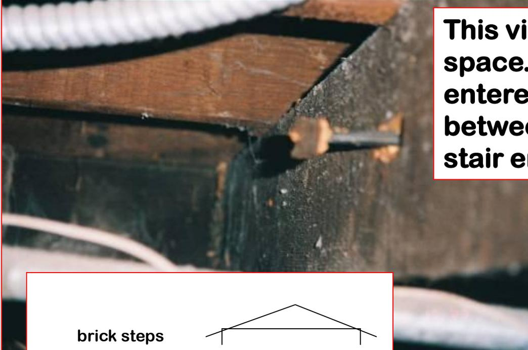
This view is of a girder in a crawl space. The rhizomorph of *Meruliporia* entered the girder by growing between the exterior wall and an brick stair entry into the home.
