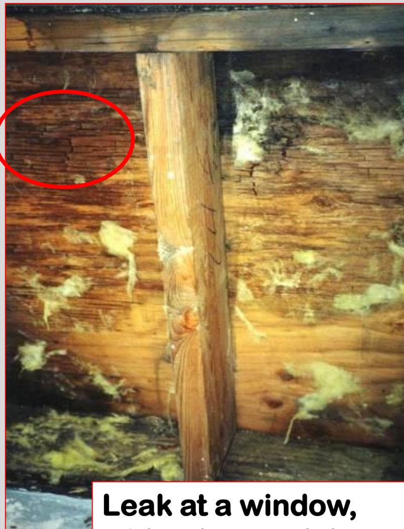
**Leak at a window, with advanced decay in plywood sheathing.**
