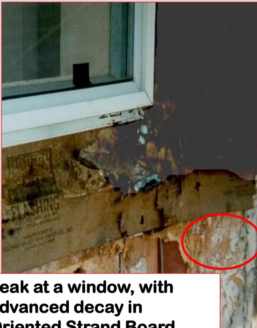
**Leak at a window, with advanced decay in Oriented Strand Board (OSB) sheathing.**
