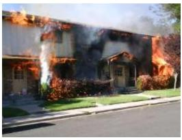
Figure 5. A cigarette thrown out the window into a 'foundation planting' of ornamental junipers burned this apartment in Reno (Photo courtesy of the University of Nevada Cooperative Extension Living with Fire program)
