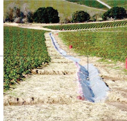
Road with a low spot in the center. Due to the steep slope, the center is covered by plastic.
