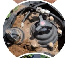
**11 Pressure regulating valve (PRV)**
