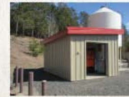
Minnesota Dept. of Natural Resources Tower, MN 440 MBH
