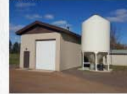
Arrowhead Regional Corrections Facility- NERCC- Saginaw, MN 4,435 MBH
