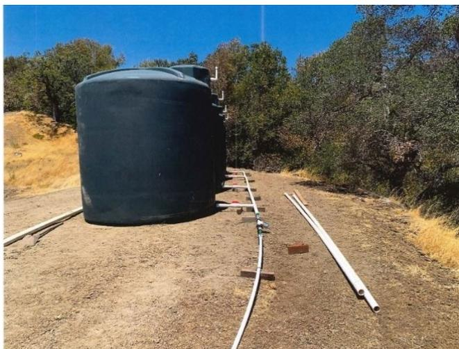
Four 3,000 gallon tanks and plumbing that form a small above ground storage system. This system can store hauled water and is also connected to on-site water sources for storage.
