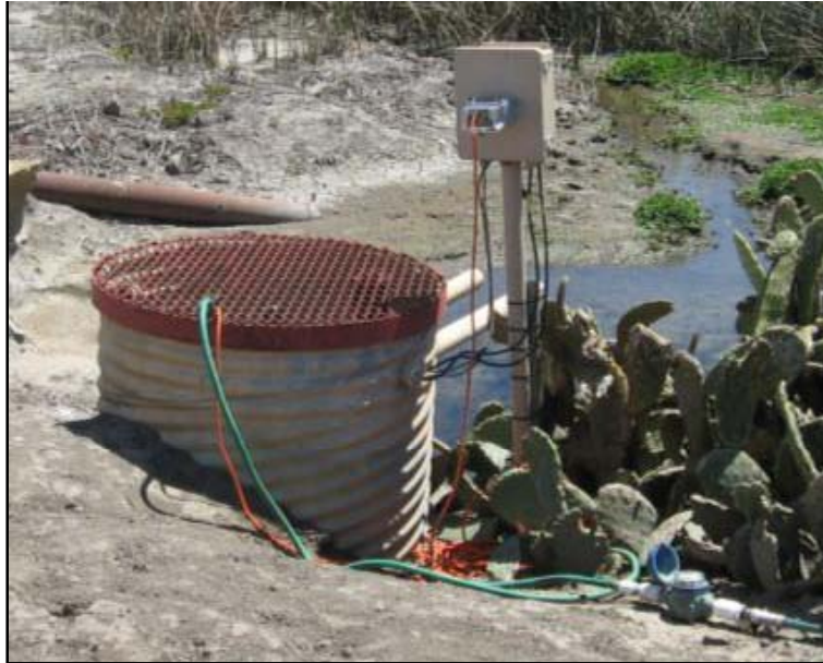
Continuous pumping into DBRs from tile drain sump or tailwater pond
