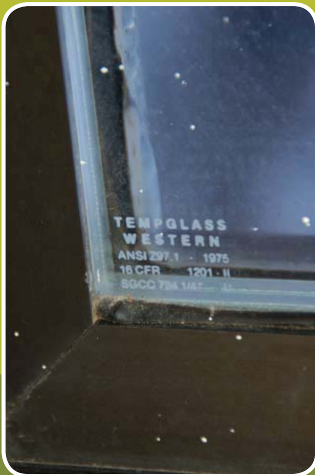
The 'bug' in the corner of this glass window pane indicates that it is tempered glass.
