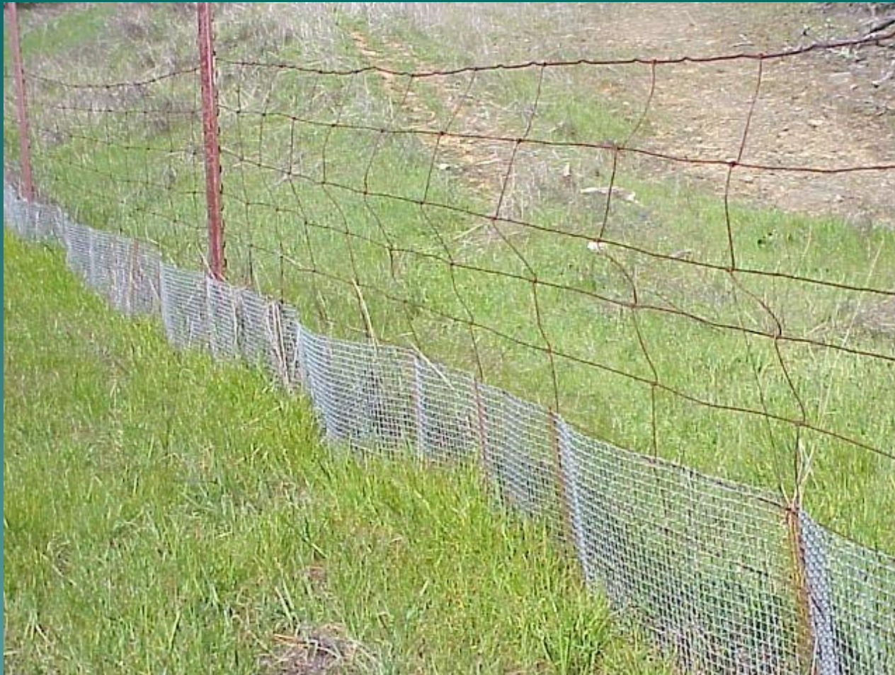
Hardware cloth attached to existing fence
