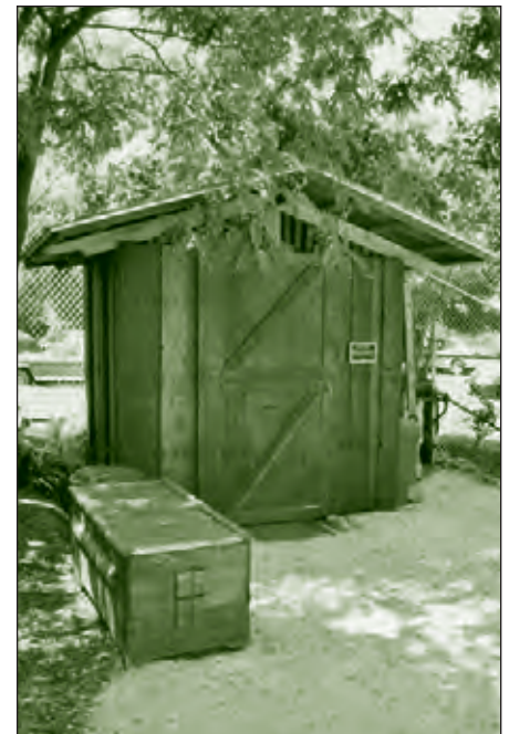
Garden shed made with salvaged lumber from deconstructed warehouses at Oakland Army Base.
