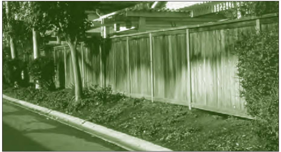
Damage to fencing from sprinkler irrigation.
