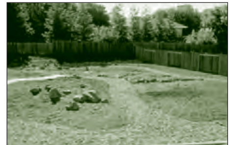
Sheet mulched site is ready for planting.
