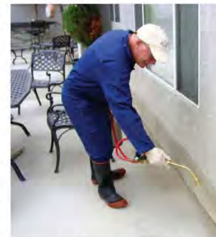
Figure 1. Applying a fan spray 1 foot up and 1 foot out from a house foundation.
