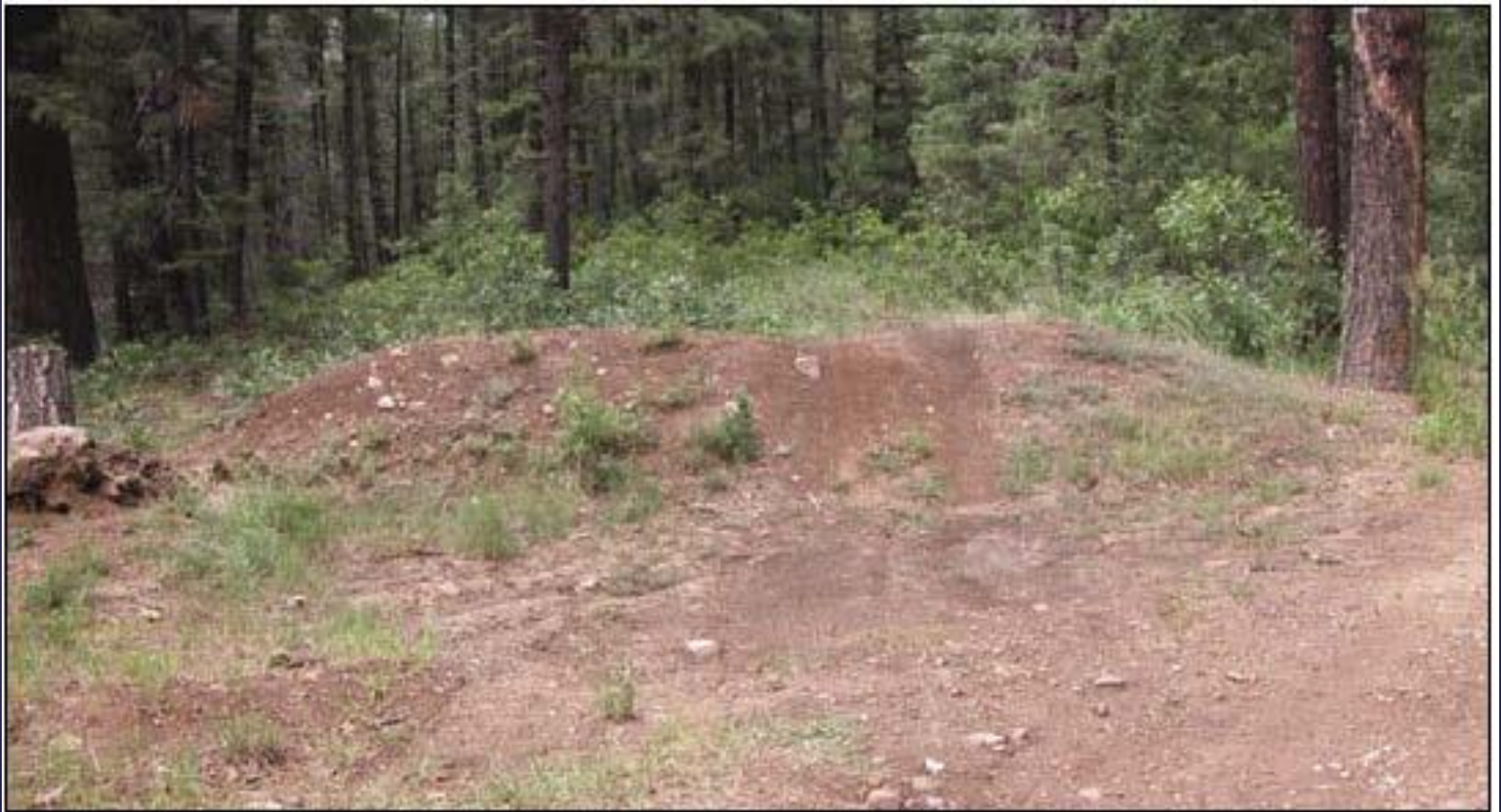
Figure 28 —Maintenance level 1 road that has been blocked to highway vehicle traffic by an earth mound.
