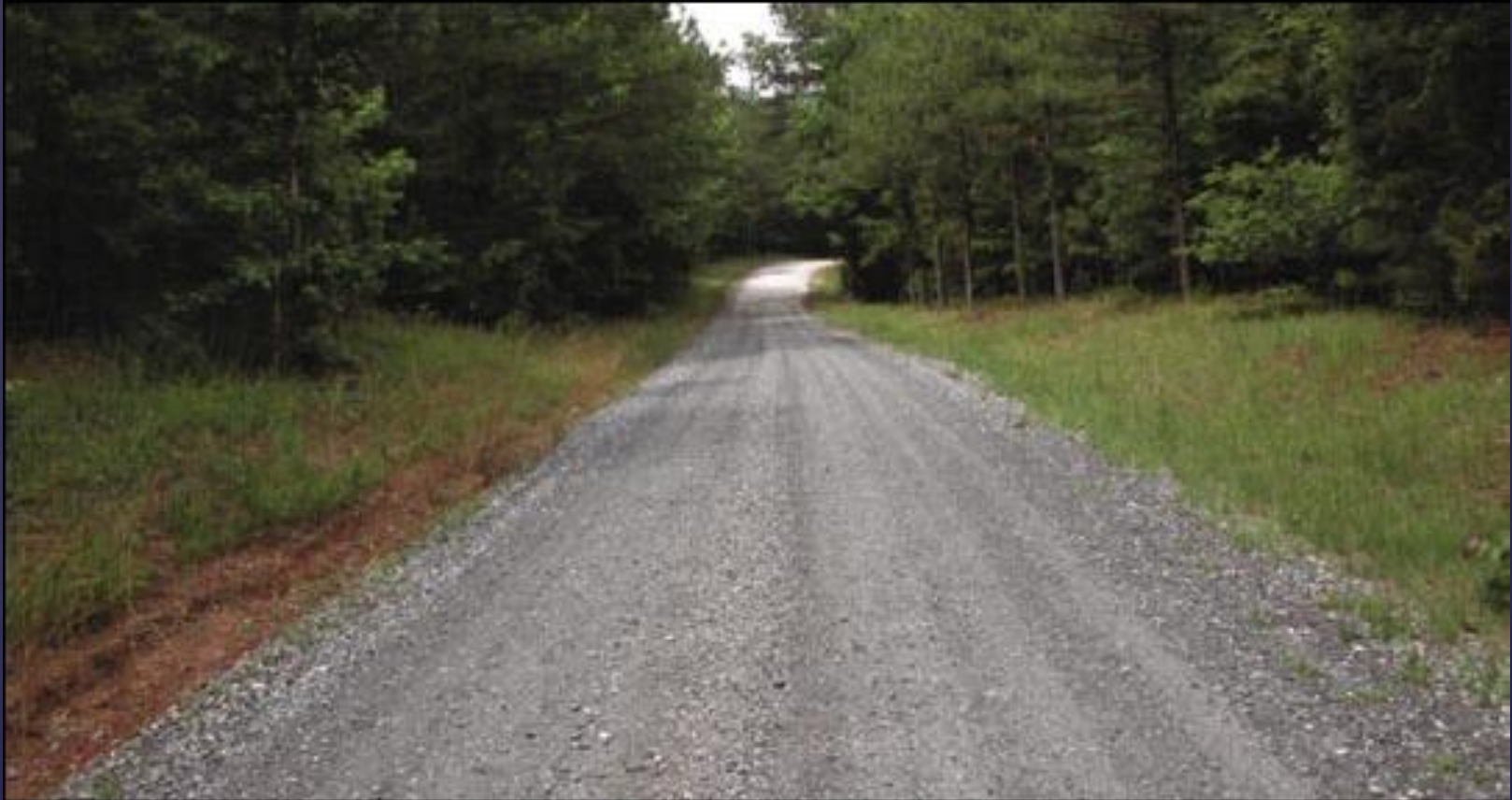
Figure 9—Maintenance level 4 road with single lane, gravel surface, and gravel shoulders.
