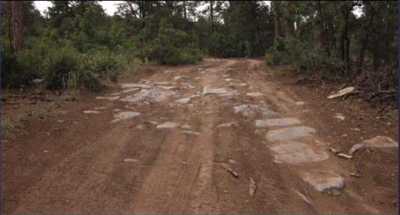
Figure 25—Maintenance level 2 road with single lane, native surface, no shoulders, and suitable for high-clearance vehicles only.
