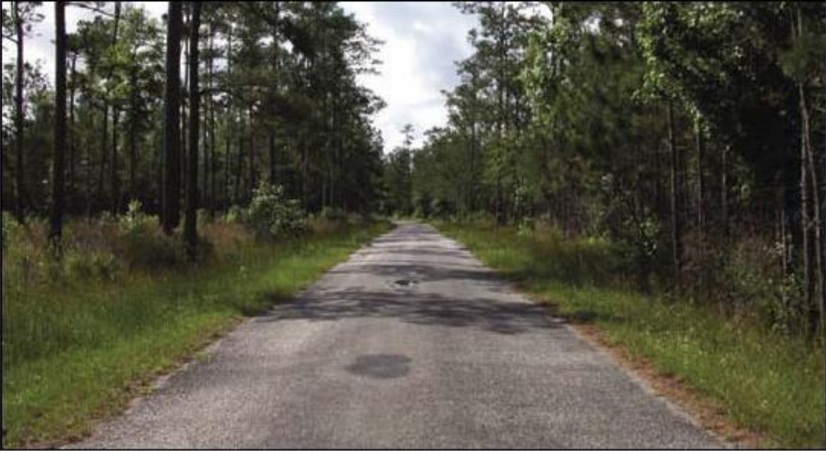
Figure 10—Maintenance level 4 road with single lane, chip-seal surface, and chip-seal shoulders.
