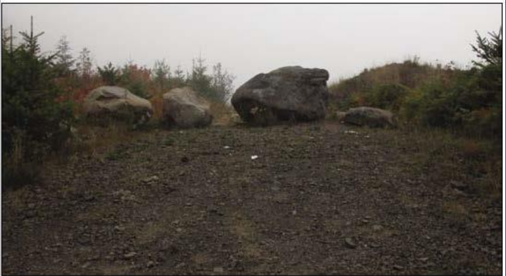
Figure 30—Maintenance level 1 road that has been blocked to highway vehicle traffic by boulders.
