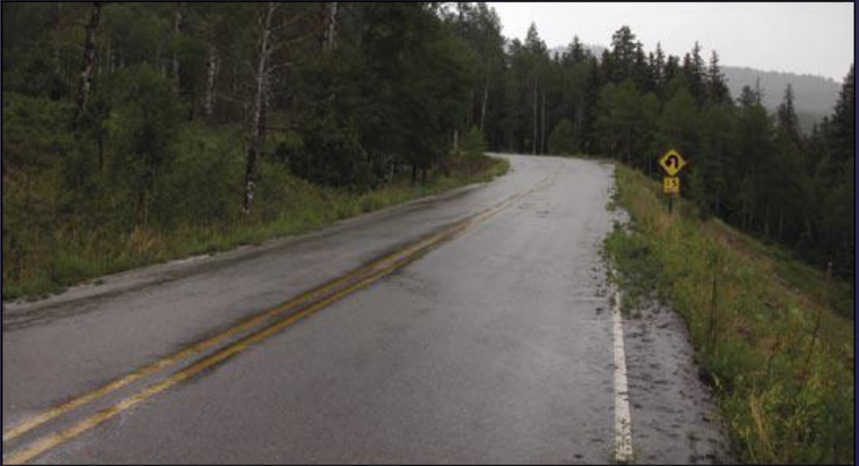
Figure 4—Maintenance level 5 road with double lanes, asphalt surface, and grass on asphalt shoulder.
