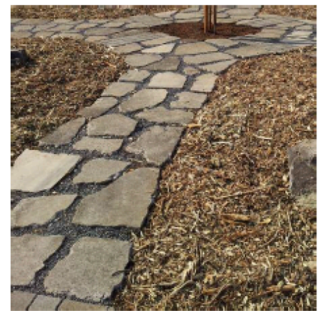
Permeable Recycled Concrete Path
