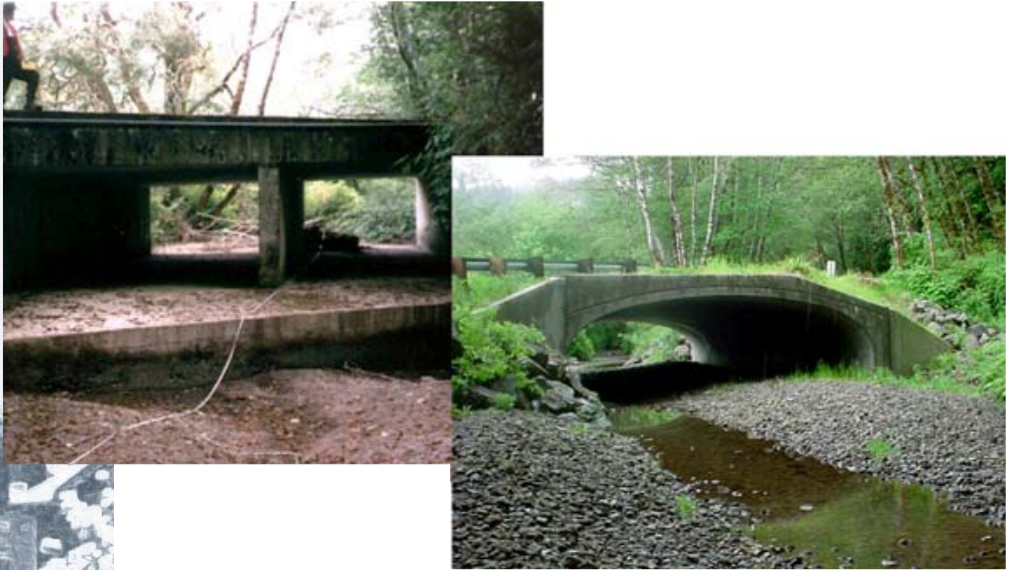
Figure 12. The double box culvert on the left was a complete barrier for all age classes of salmonids on Minot Creek in Northern California due to stream velocity, depth, and leap height. It was replaced by the bottomless concrete arch culvert on the right. The project opened up 2.5 miles of upstream habitat to salmonids. Source: Courtesy FishXing, http://www.stream.fs.fed.us/fishxing/case/ .
