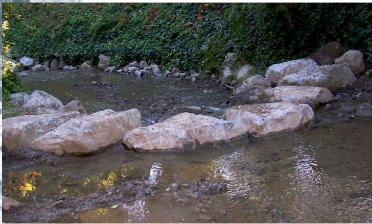
Figure 21. This rock weir has been installed to absorb the energy of the stream and reduce its ability to erode the banks. This helps reduce the need to install other bank-hardening measures that would impair aquatic habitat. Photo: R. Harris.
