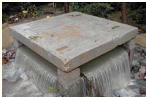
Figure 34. An outfall weir disperses storm water into a shallow area for infiltration. Photo: Deven Lindenberg, BLWI.
