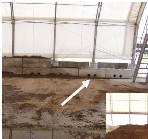
Aeration pipe connections to blowers behind block wall
