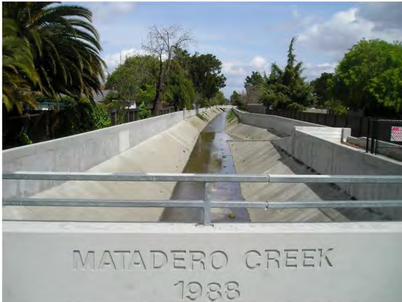
Concrete Lining with Floodwall – Matadero Creek
