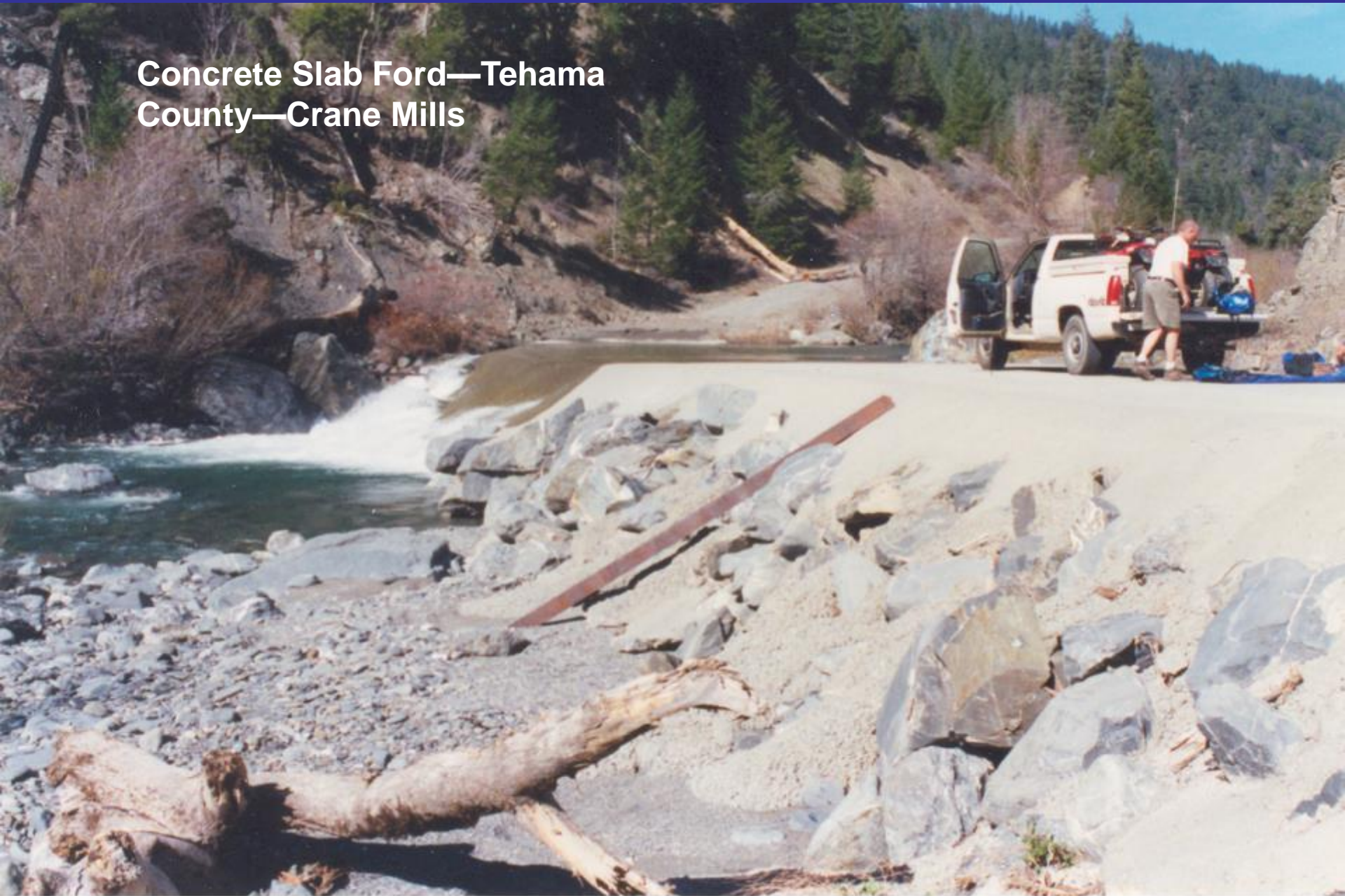
Thomes Creek "The Slab."
