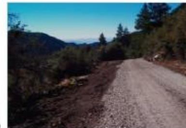
Figure 1. Low-volume road that has been newly graded and out-shaped. San Bernardino County, Advisor Richard Harris.
