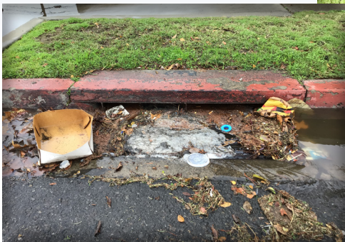
Below: Storm drain inlet clogged with leaves and debris.
