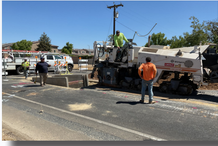
Pavement grinding to begin trenching for the storm drain on Armstrong
