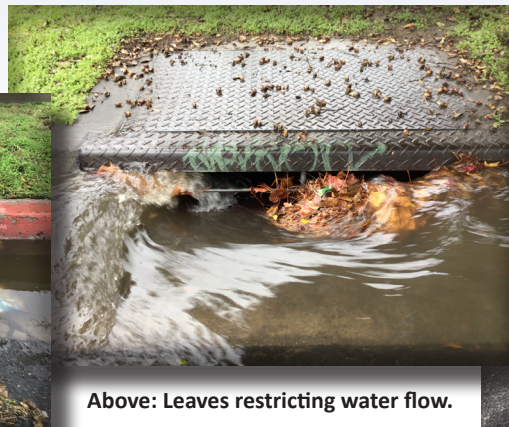
Below: Storm drain inlet clogged with leaves and debris.
