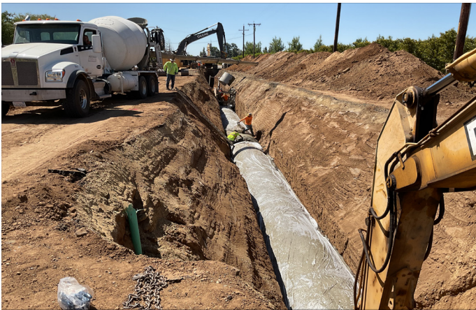
BS-26: 60 Inch cast in place storm drain construction on Armstrong
