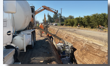
66 Inch cast in place storm drain pour on Armstrong
