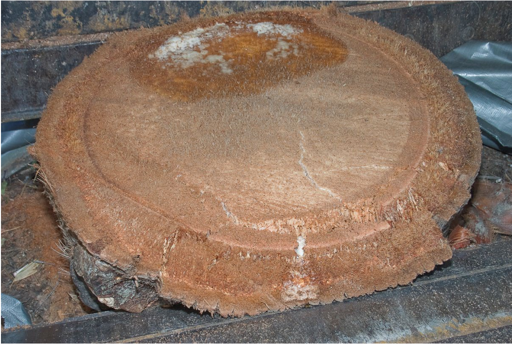
9. Cross section of base of trunk of Mexican fan palm with suspected Ganoderma zonatum showing internal discoloration and decay (top), Pasadena, California. © 2010 D. R. Hodel.
