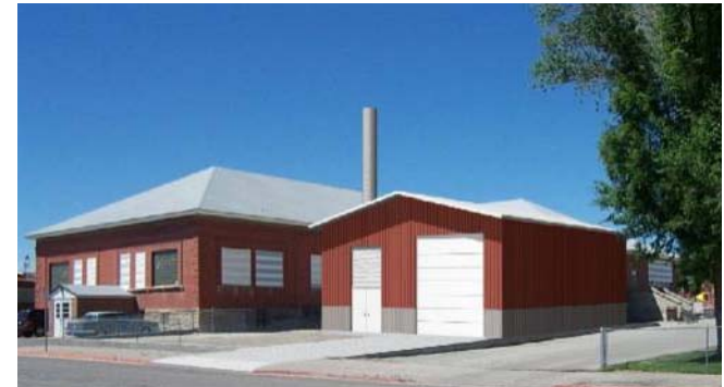
Boiler house and School, Ely NV
