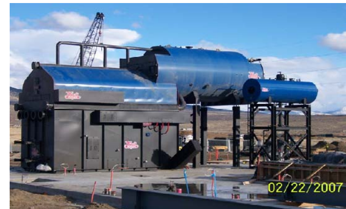
Boiler Installation, Correctional Facility Carson City, NV
