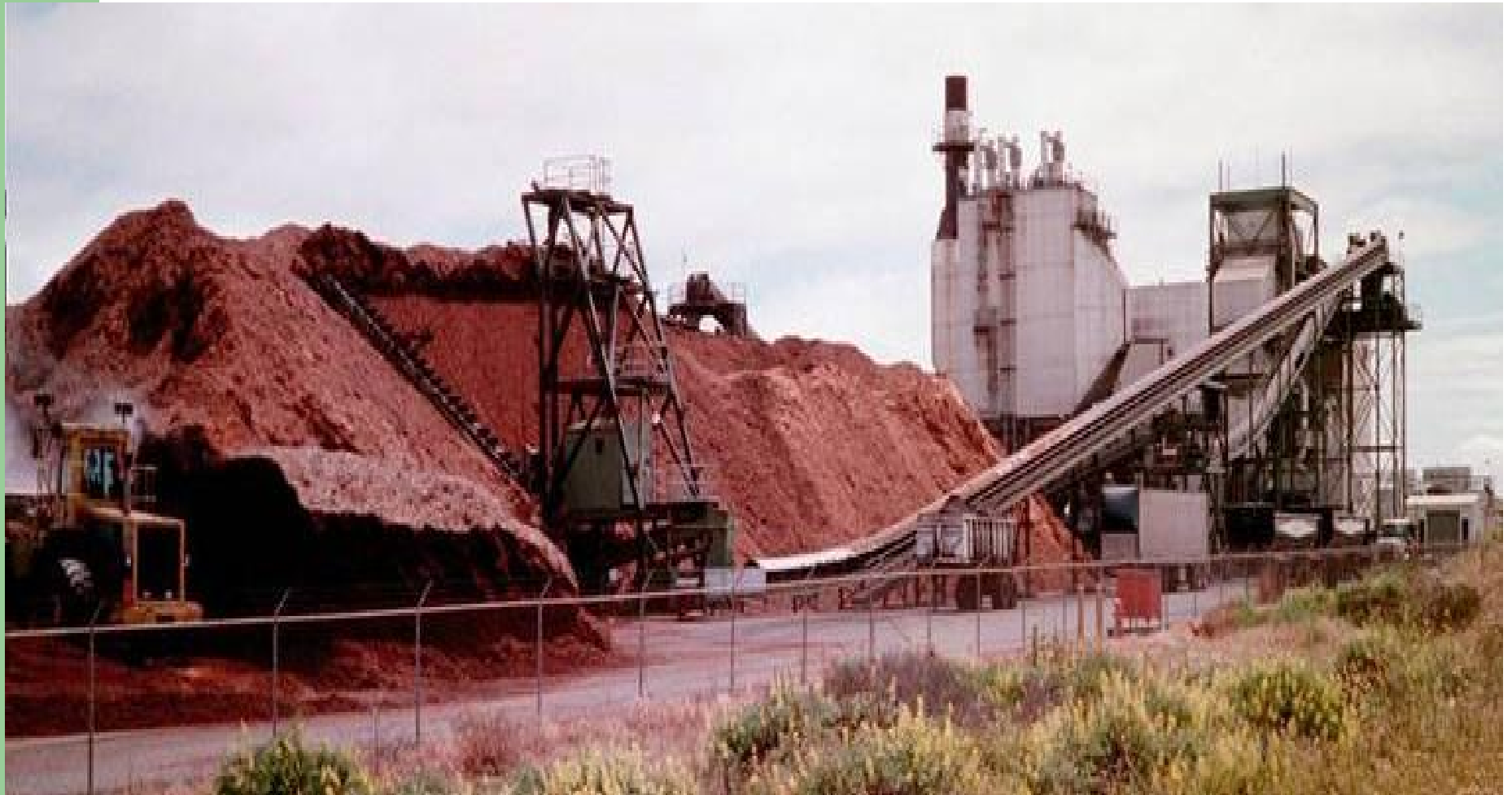
DG Fairhaven Power 18 MW CHP at Fairhaven
