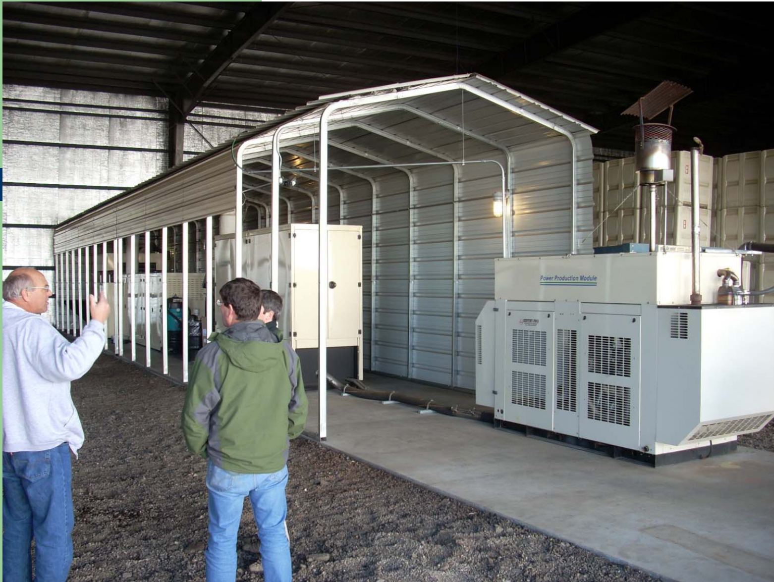
Community Power Corp BioMax 50 kWh CHP at Dixon Ridge Walnut Farm, Winters
