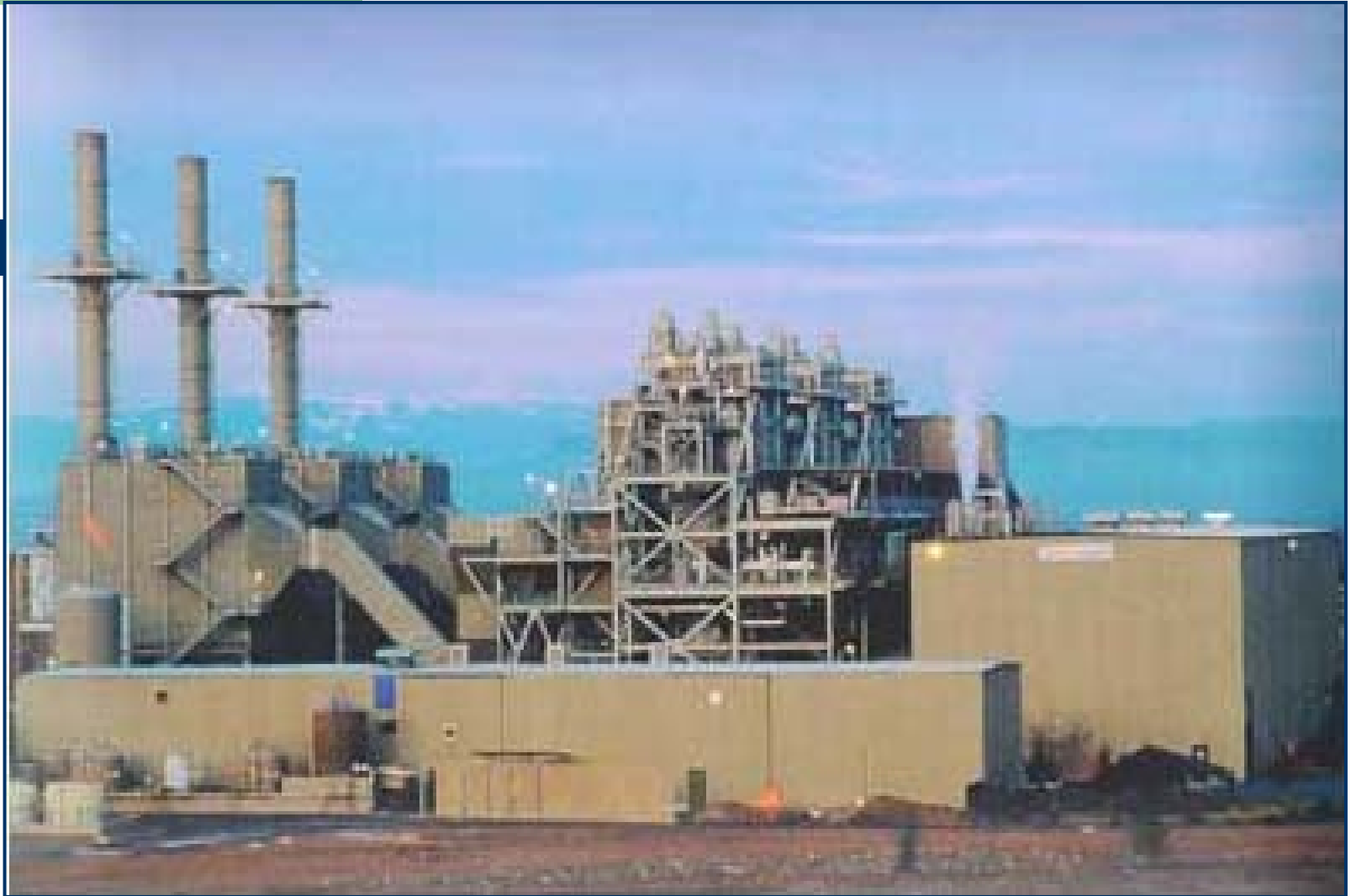
Wheelabrator Shasta Energy Company 50 MW Generation facility at Anderson
