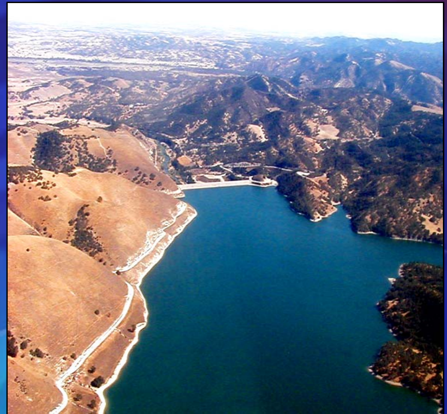
San Antonio Reservoir Completed in 1967 Lake Capacity 335,000 AF
