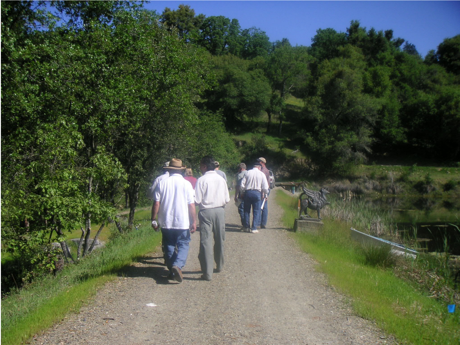
Note repair to erosion on top of dam.
