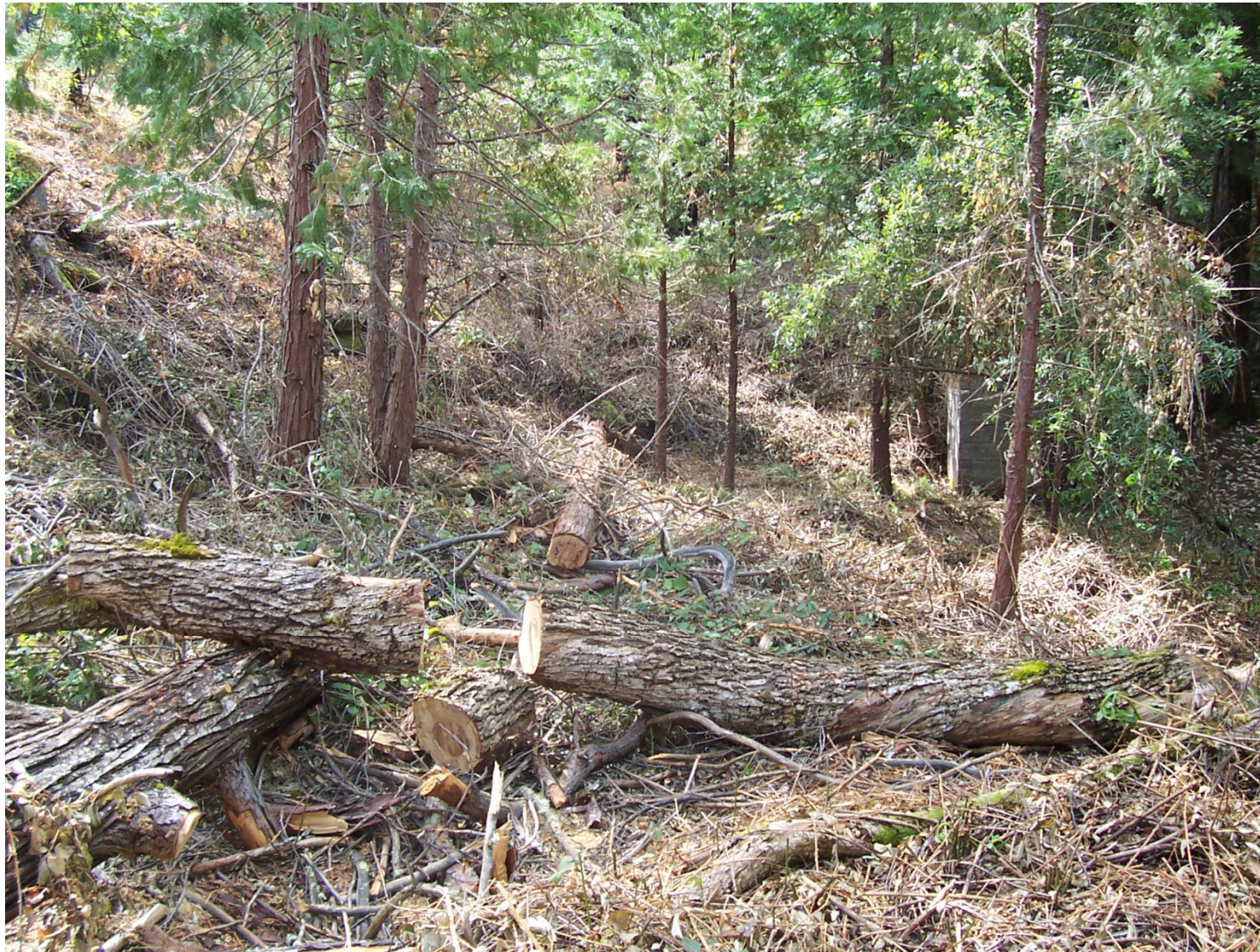
View of downstream face of embankment toward pump house. (8/16/05).
