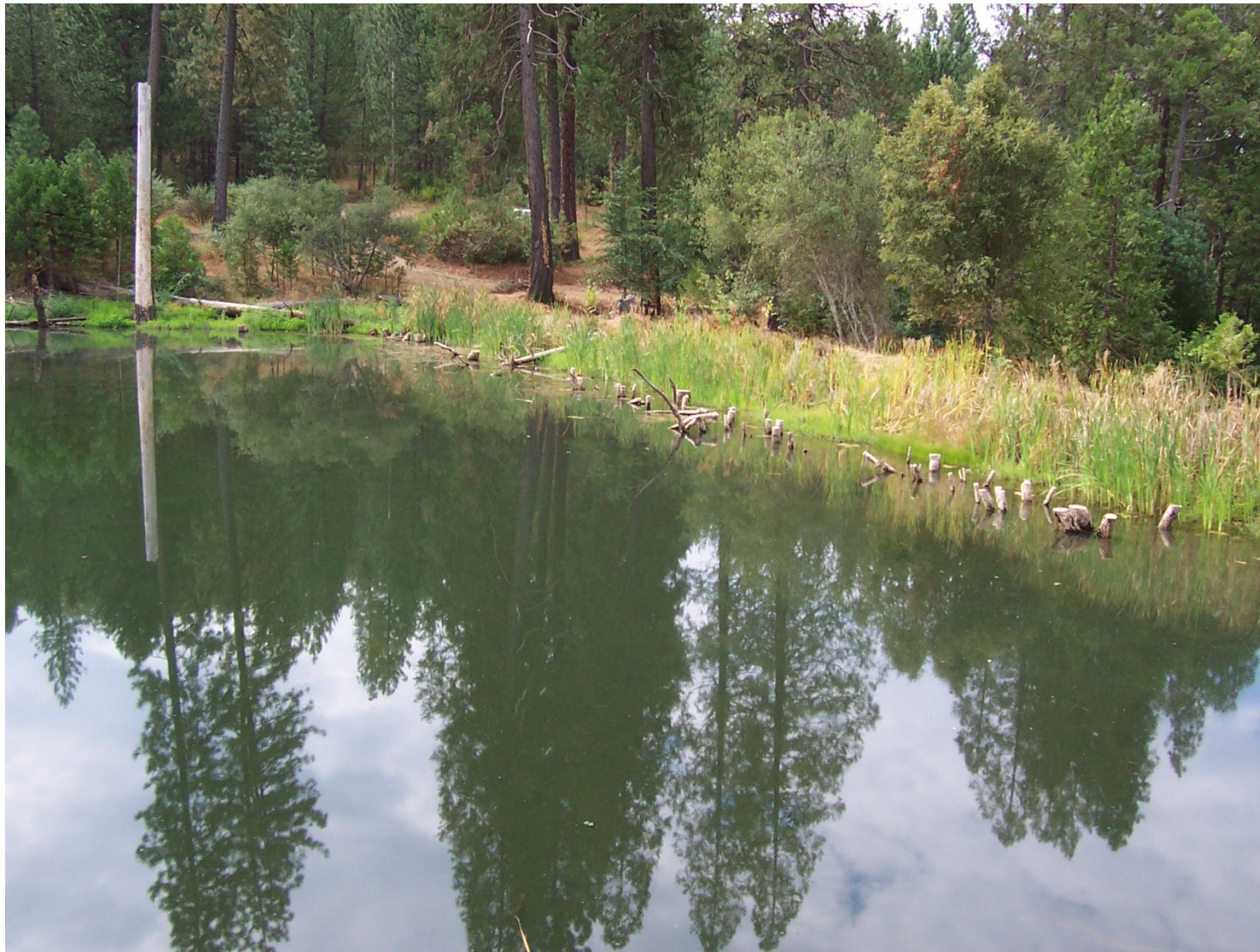
View of embankment from north side of reservoir (8/16/05).
