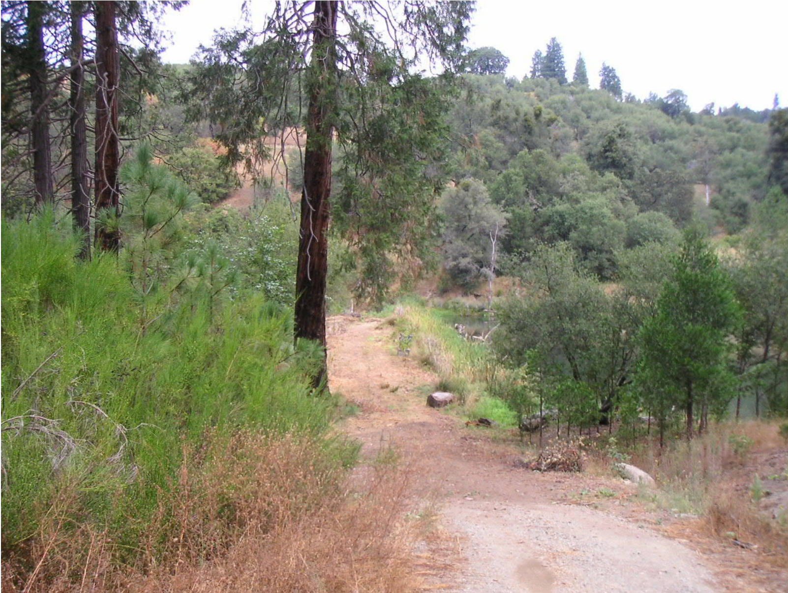
Top of Dam looking toward emergency spillway.
