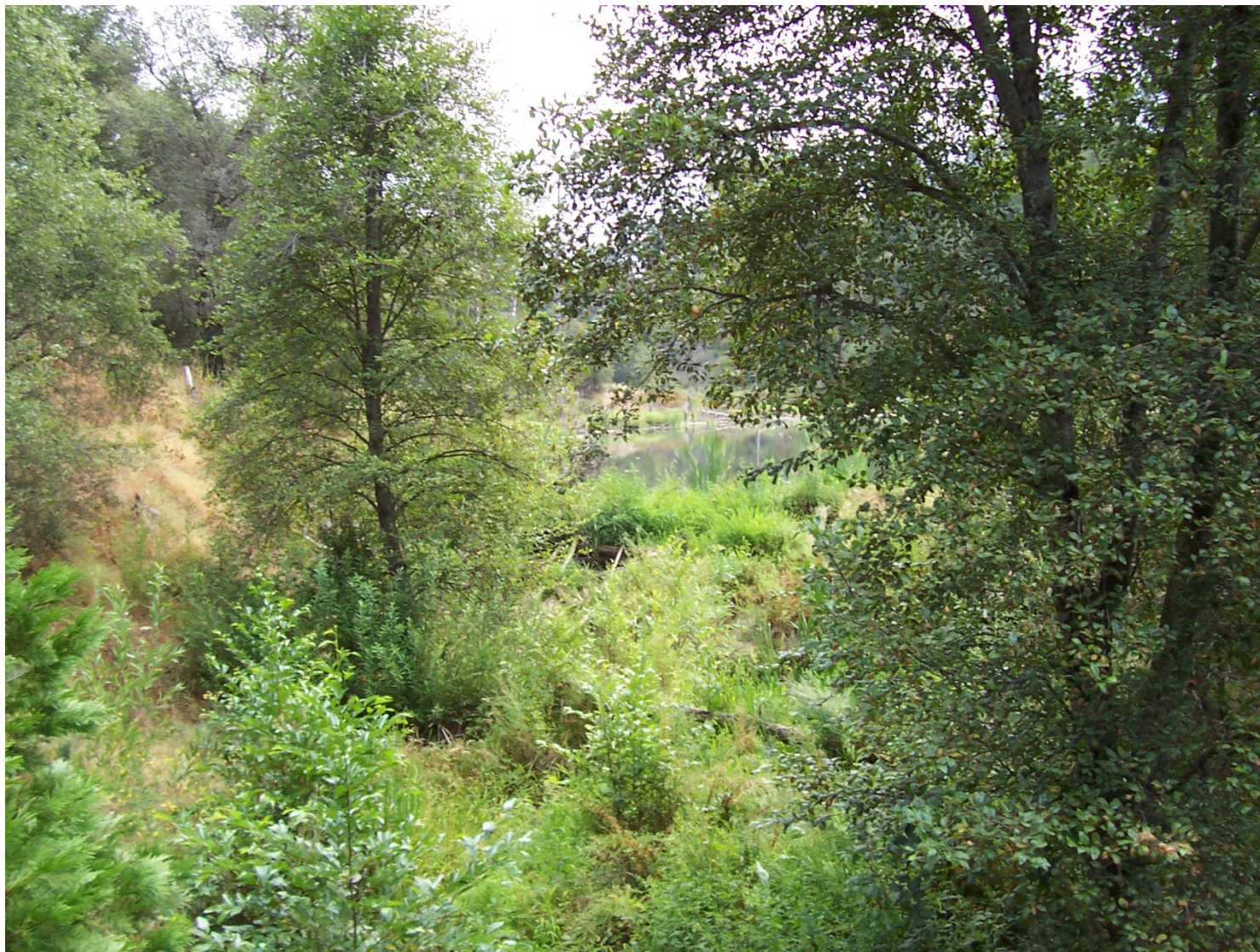
View upstream at vegetation in emergency spillway exit channel (8/16/05).
