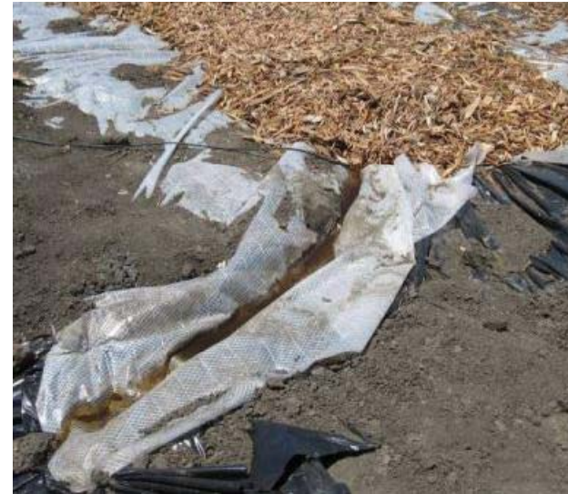
Outlet drains into surface ditch after approximately 2 days residence time
