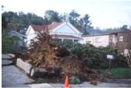
incense cedar root failure
