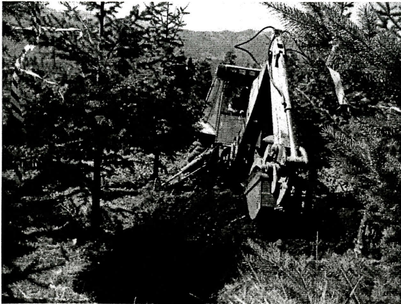
Site 1 – Douglas-fir - Back hoe begins digging
