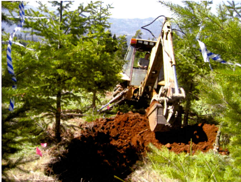
Site 1 - Douglas-fir - Back hoe begins digging
