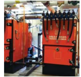
A biomass thermal system can provide hot air, water, and process heat
