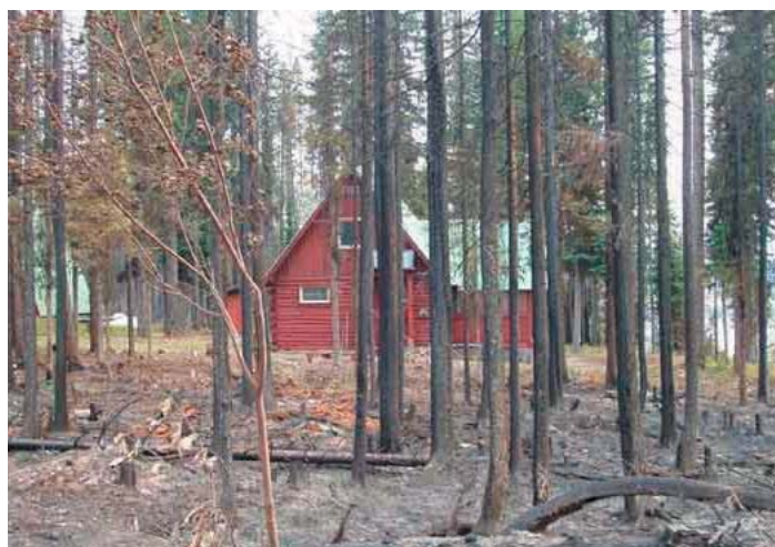
Sound fire prevention techniques saved this house.
