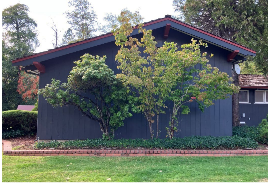
Figure 26. Existing condition, Area 8, unmodified photograph, September 2025.
