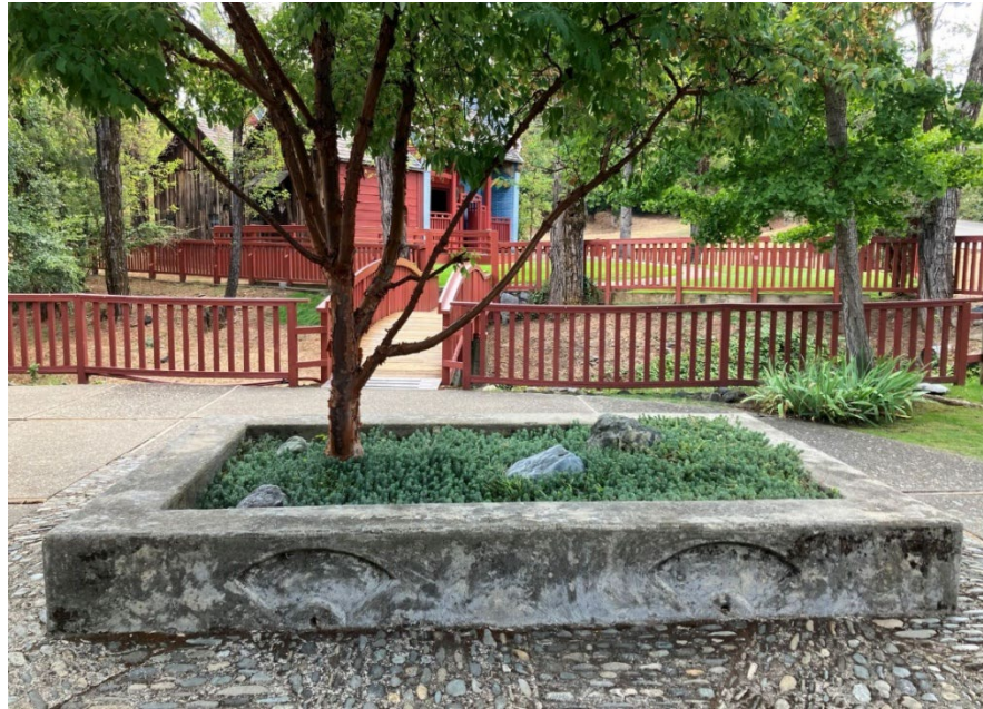
Figure 11. Existing condition, Area 4, unmodified photograph, September 2025.
