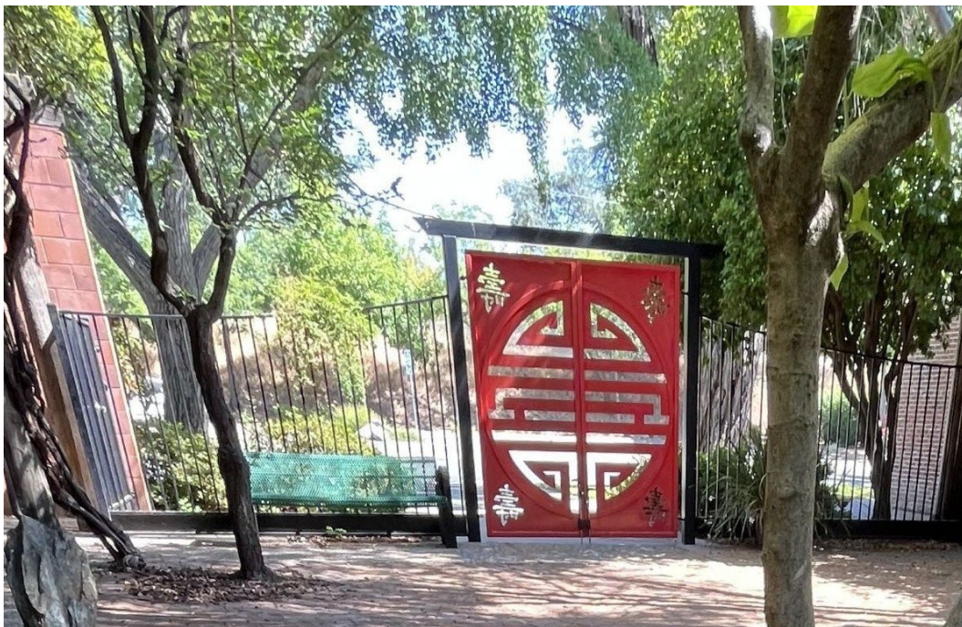
Figure 35. Black steel fence and red steel gate, Oroville Chinese Temple, June 2025. 11
