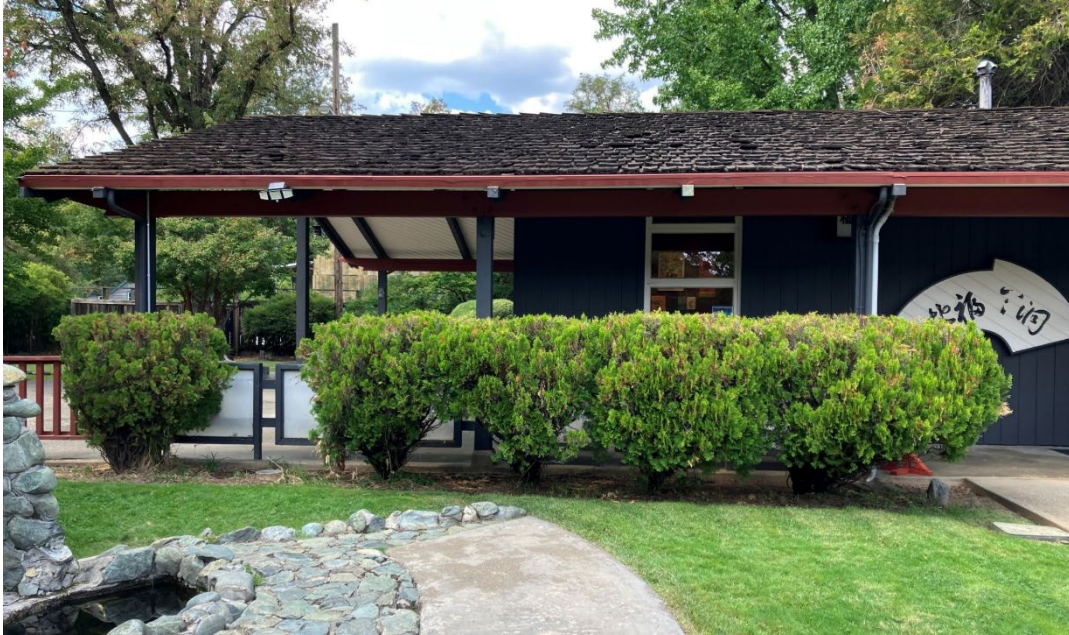
Figure 5. Existing condition, Area 2, unmodified photograph, September 2025.
