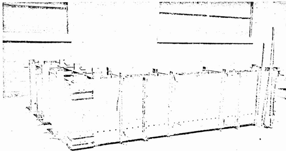
FORMS for rammed earth construction, showing the arrangement for forming corner and partition walls and for blocking out openings. The spacing of the bolt holes along the bottom of the form permits adjustment to all wall thicknesses that are divisible by 3". Three types of hand-tamping tools are shown in the photograph at the far right.
