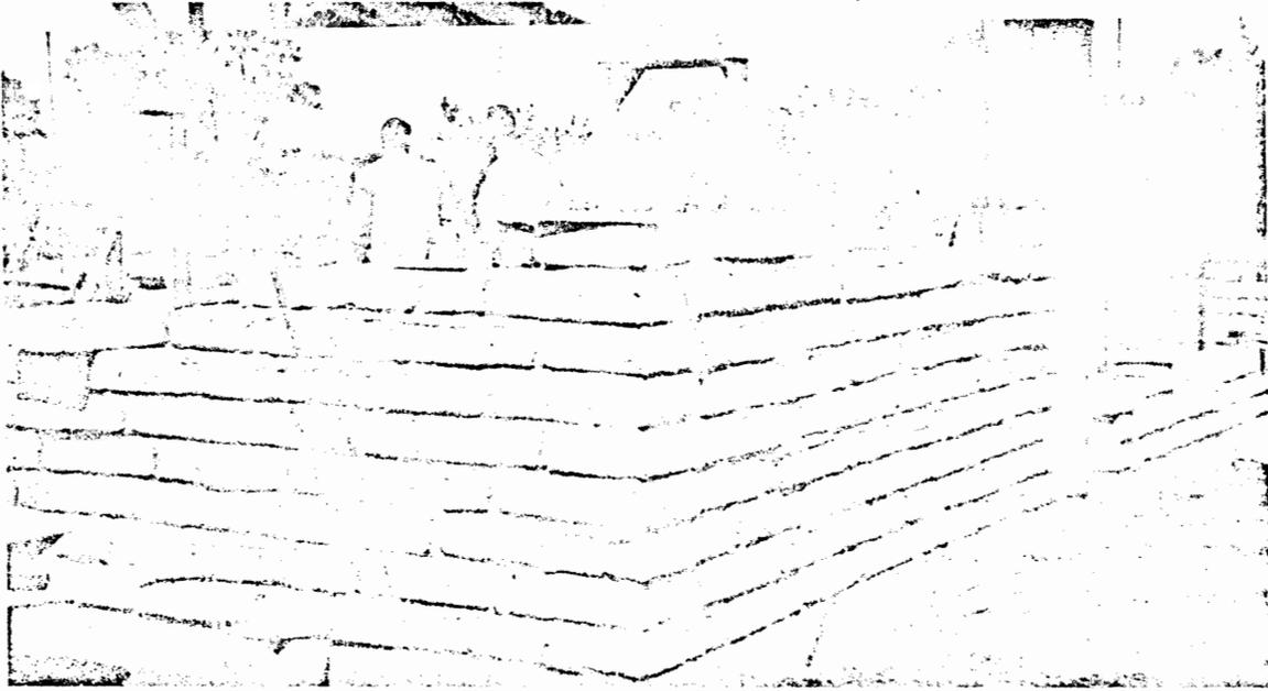
ADOBE-HOUSE CONSTRUCTION, showing brick arrangement, vertical reinforcing steel, and door frames in place.
