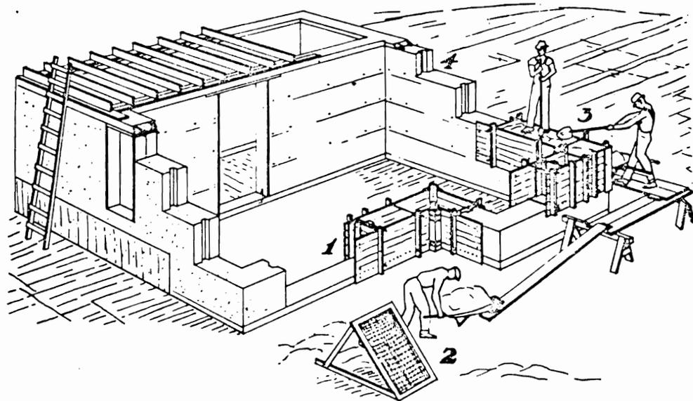
RAMMED-EARTH WALL CONSTRUCTION. Heavy sectional forms are clamped to the masonry foundation (1). Damp soil is put through a coarse screen (2) and is spread 4 inches thick in the forms (3). This is tamped to a dense mass, and the routine continued until the form is full. Cross-bolts are then withdrawn and the forms moved. Vertical joints are staggered at least 3 feet, and shaped with tongue and groove (4). A reinforced concrete bond beam is poured along the top of the wall.
